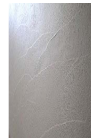
漆喰塗布状況
