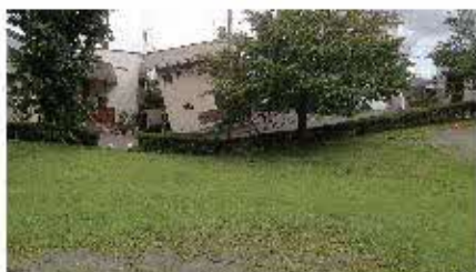
第19図 凹地状地盤陥没と傾動した家屋(里塚北西部)。 Fig. 19 Depression of ground surface and tilted house at northwestern Satoduka area.
