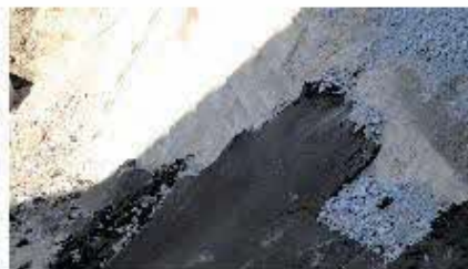
第16図 地溝状亀裂の壁面に現れた埋没擁壁。 Fig. 16 Buried retaining wall at the side wall of graven-like clacks, right bank of Omagari river.
