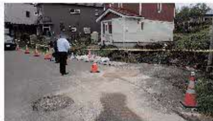
第15図 地溝状亀裂周辺で発生した噴砂。 Fig. 15 Sand boil from the crack near the graven-like clacks, right bank of Omagari river.
